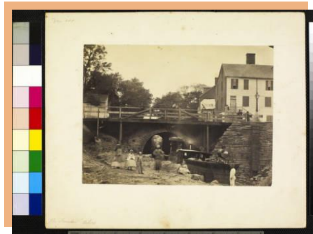
The Wythe Street tunnel
